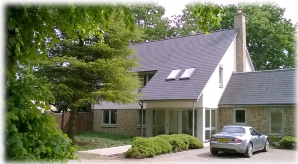
March Vicarage, 177 Station Road, March.
